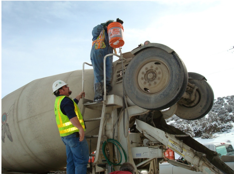
Fig. 4. TOXECON™ ash added during concrete mixing.
