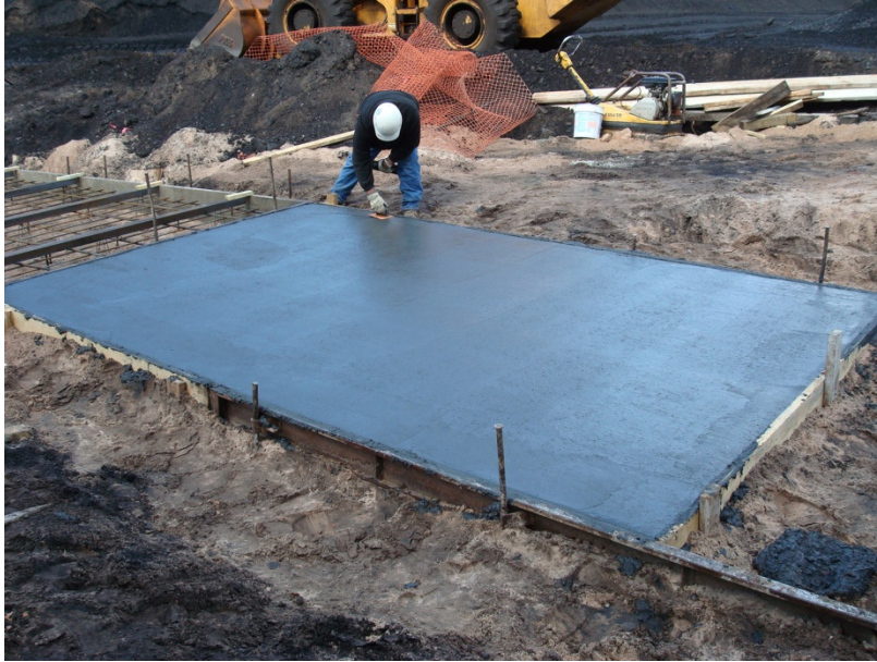
Fig. 8. First successful high-carbon concrete placement.
