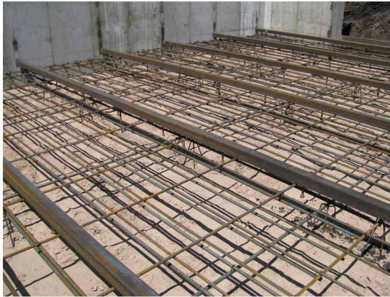
Fig. 6. Completed push wall and support steel for high-carbon concrete pad.
